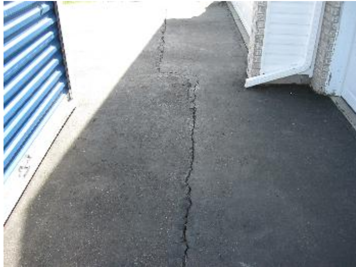
Grounds Driveway condition
